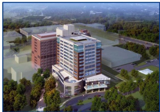
Figure 2: Exterior rendering showing the circular entrance and precast concrete façade (Provided by Turner Construction)
